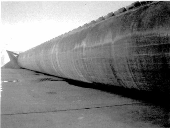
PHOTO NUMBER: 15 PHOTO DIRECTION: North DESCRIPTION: Along the downstream side of bladder #2.
