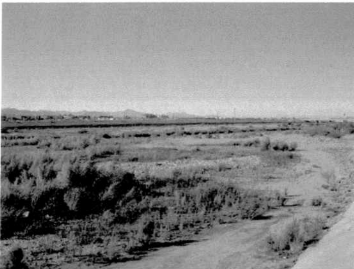
PHOTO NUMBER: 7 PHOTO DIRECTION: West DESCRIPTION: Toward downstream as seen from above the right abutment or north side of the river bank.
