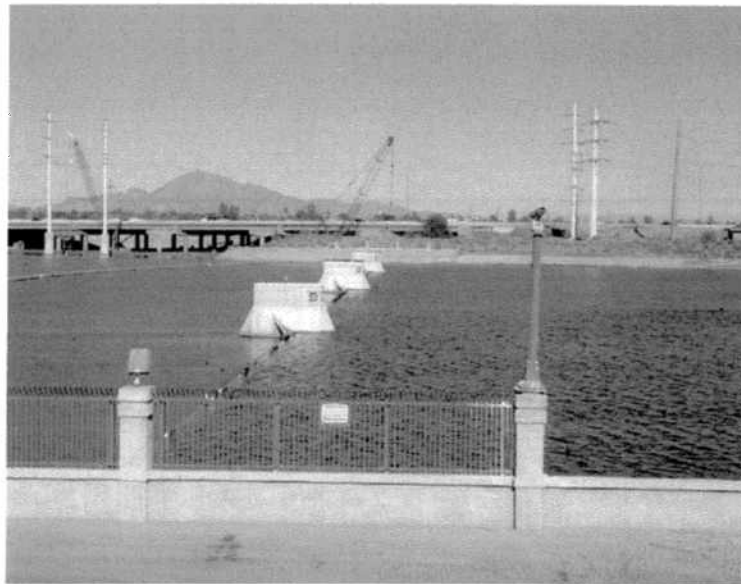
PHOTO NUMBER: 23 PHOTO DIRECTION: North DESCRIPTION: View of the nearly submerged upstream dam as seen from the south bank.
