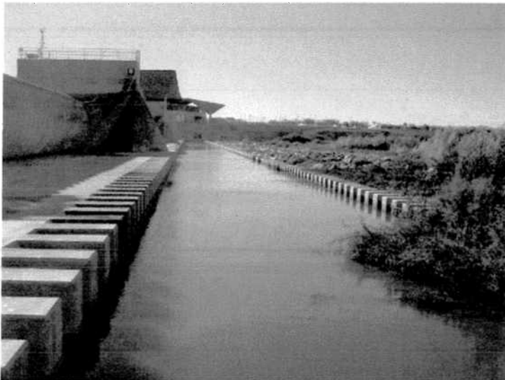
PHOTO NUMBER: 9 PHOTO DIRECTION: South DESCRIPTION: Another view along the stilling basin and foundation slab from the right abutment.
